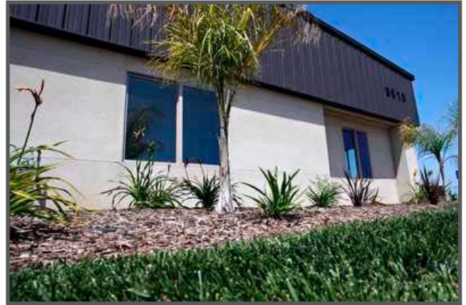
A new smaller industrial office building at Nicholas Plaza in Visalia is an example of Pickett & Sons' work. The company is having success with these smaller structures as the vacancy rate drops in Fresno and Visalia.
